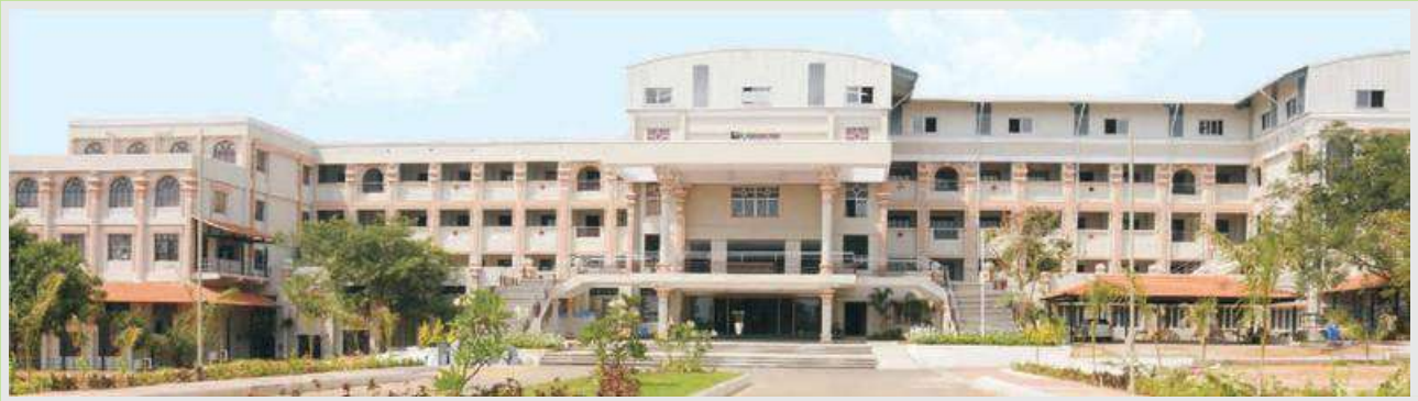
PMC TECH - Engineering Main Block
