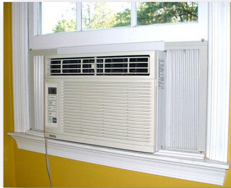
Window Air-Conditioning System
